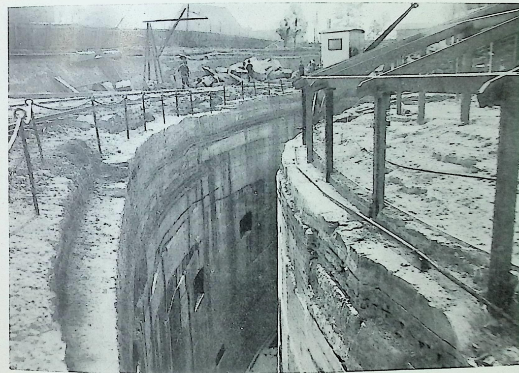
TRENCH MADE BY "SISKOL" MACHINE.
