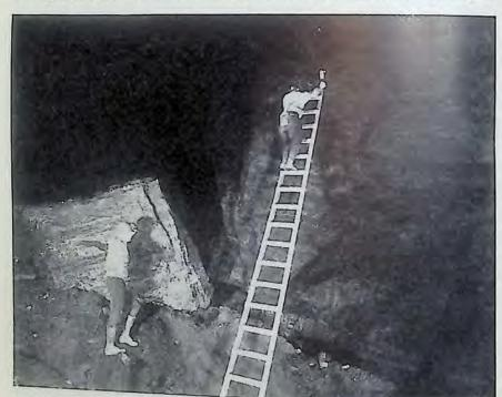
Testing for gas in Hanna No. 4 Mine. Note large block of coal shot from top mining.. This coal was mined to a height of twenty-six feet.
