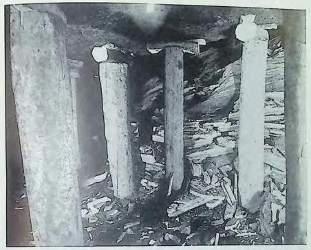
How the top caves with removal of pillars in the Rock Springs field
