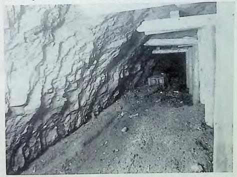
Long-wall face cut by machine for Vulcan Scrapers. Note overhang of timbering.
