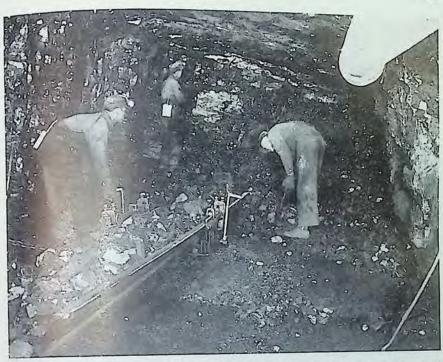
View of low type Duckbill in Rock Springs District, driving narrow work with blower pipe for ventilation. This device is now built by the Goodman Manufacturing Company, Chicago.
