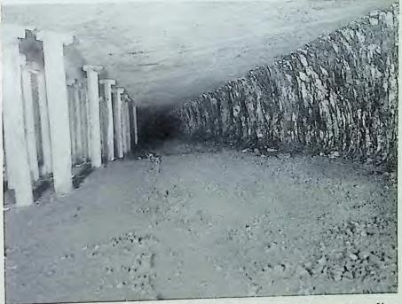
A Vulcan Scraper place cleaned up and ready for cutting machine. Note splendid roof and fine timbering.
